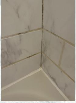
This picture shows mold in the grout lines of a shower stall. To clean this, use a disinfectant solution (i.e., bleach) and a scrub brush, or use a disinfecting wipe.
